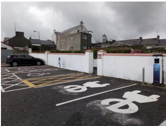
Photo No.3 – Existing wall at town car park to be demolished and replaced.
