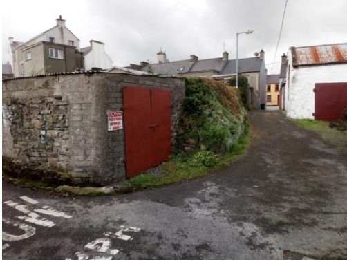
Photo No.5 – Back Lane Looking to Bridge Street
